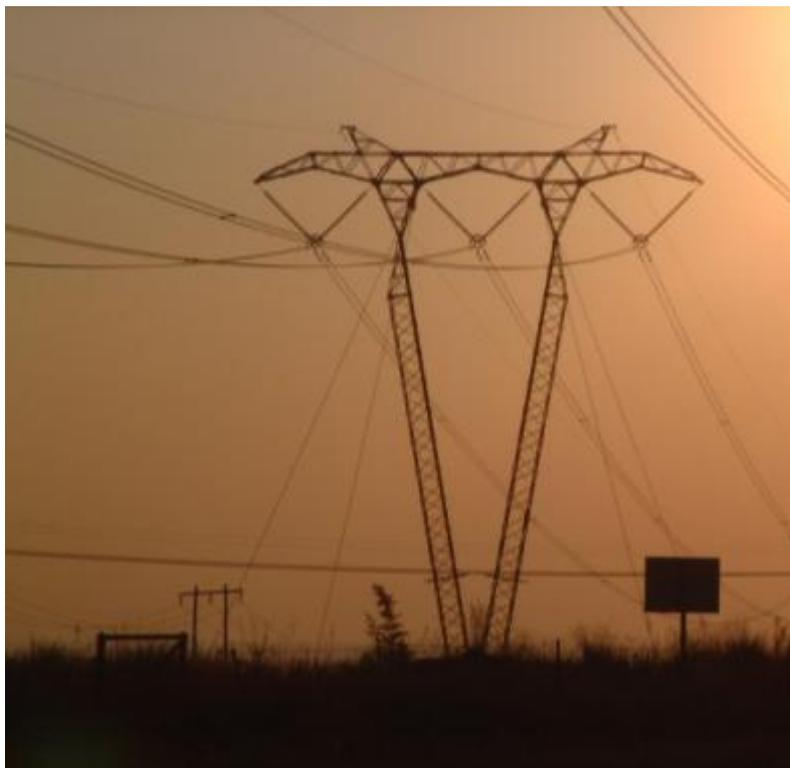
**Figure 15:** Guyed suspension tower
