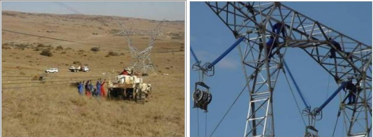
**Figure 29:** Stringing with pilot tractor (top) and pulleys (bottom)
