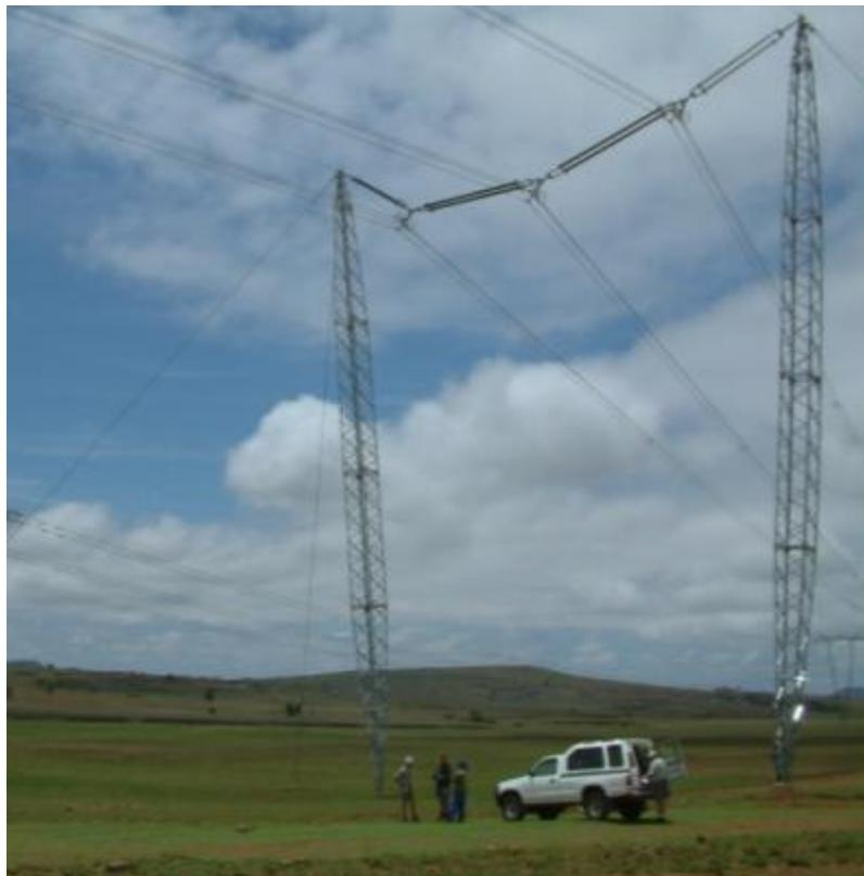
Figure 13: Cross-rope suspension tower
