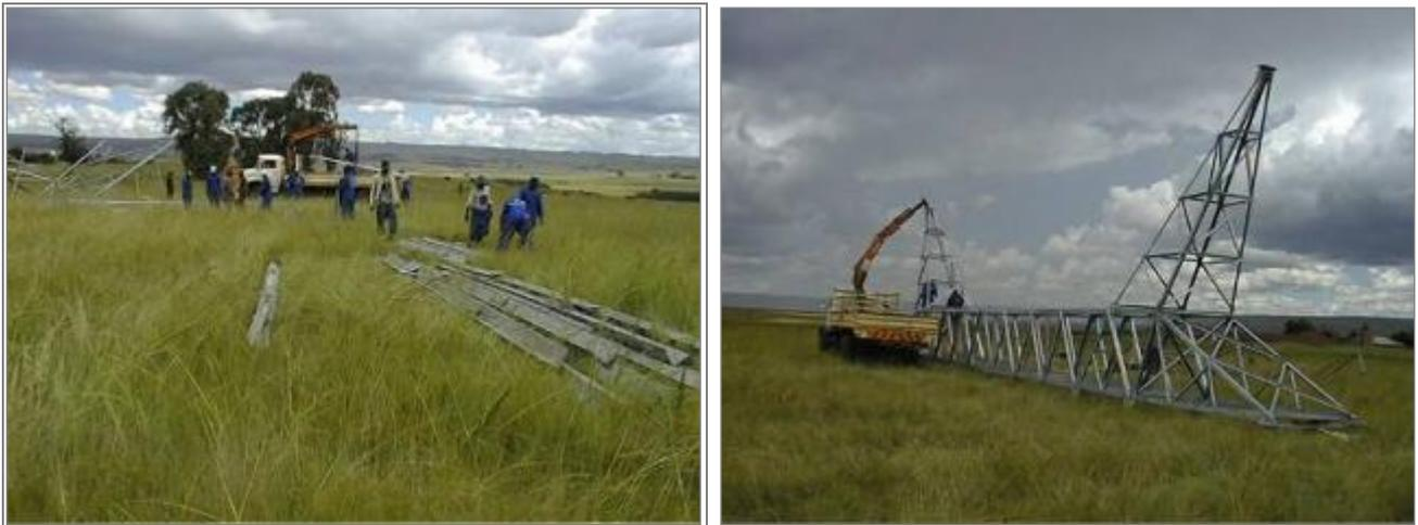
**Figure 26:** Delivery of steel (top) and assembly of tower (bottom)
